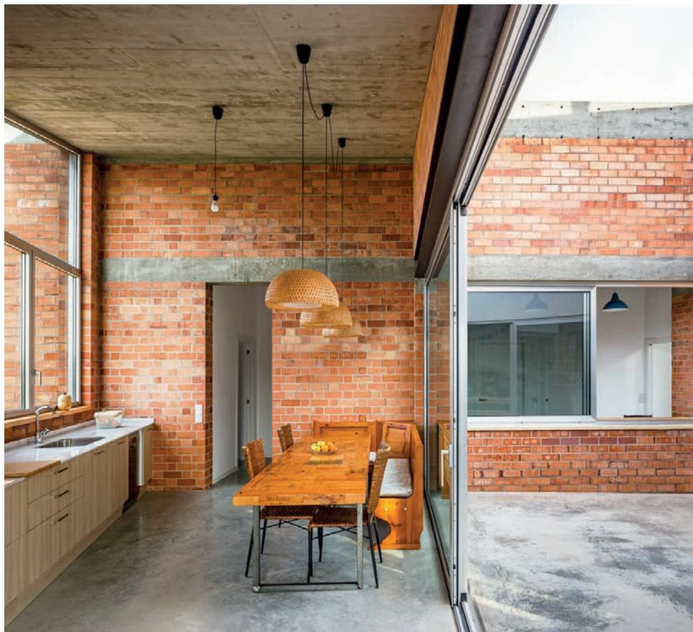
**VOLUME I** Beyond the routes, each room in the house has been built independently, piece by piece, working on sloping roofs that give each room of the house a different expressiveness. The roofs are made of concrete and have been maintained with all their visible history: formwork line and imperfections of the work process.
